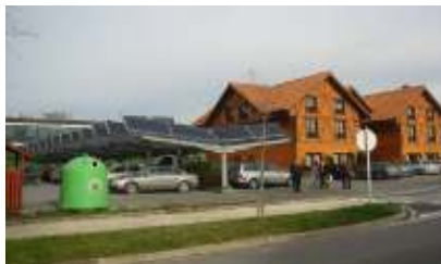
Model: LT 03 * 1 Nos Heat Source : Solar Panels
